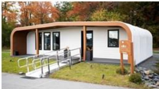
Pictured (Right): Factory of the Future 1.0. Pictured (Left): A home produced by the world's previous largest 3D printer. Source: UMaine Advanced Structures and Composites Center Facebook page.
